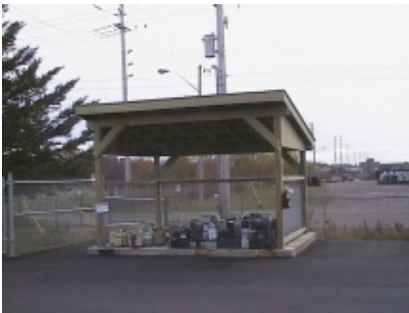
Propane Tank and Car Battery Storage Area (Southeast Corner of Site)
