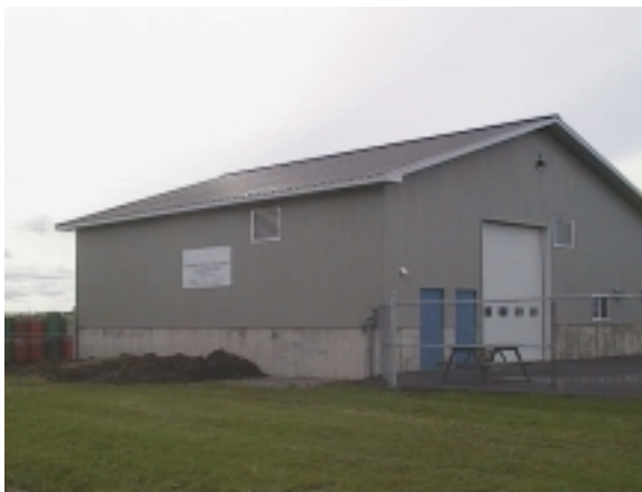
East Side of HSW Building (Landscaping to be completed Spring 2002)
