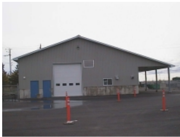
North Side of HSW Building
